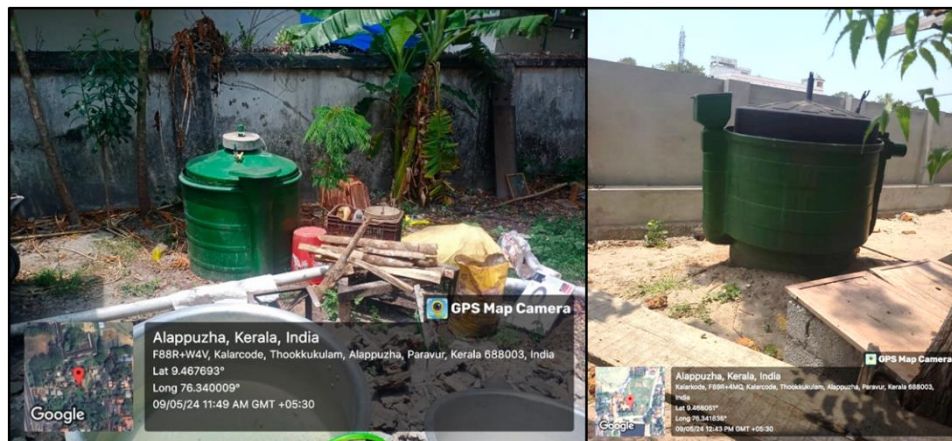
Biogas Plant observed in the campus
