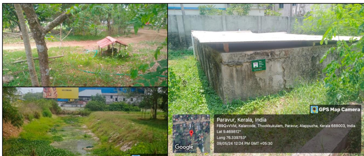
Rainwater Harvesting Unit, Pond and Bore wells observed in the campus
